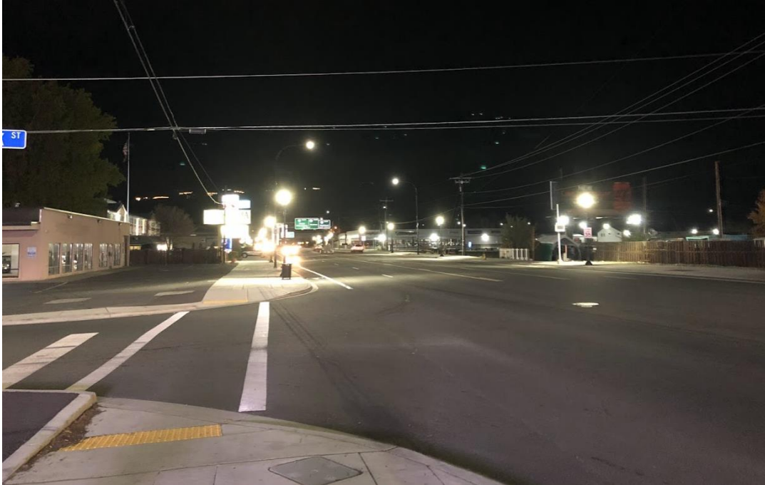
Figure 2 - North First Street in Yakima
