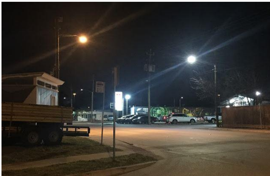
Figure 2 - HPS point source on the left, LED surface source on the right
