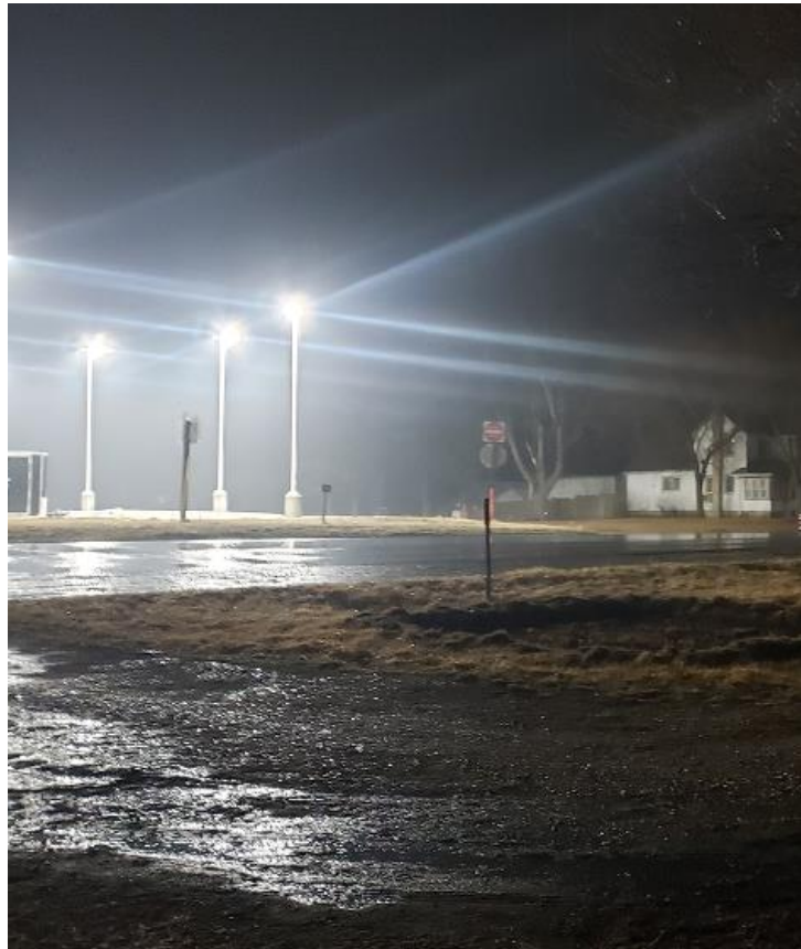
4 5 6 7 8 9 10 11 12 13 14 15 16 17 Figure 9 - LED Parking Lot Lights
