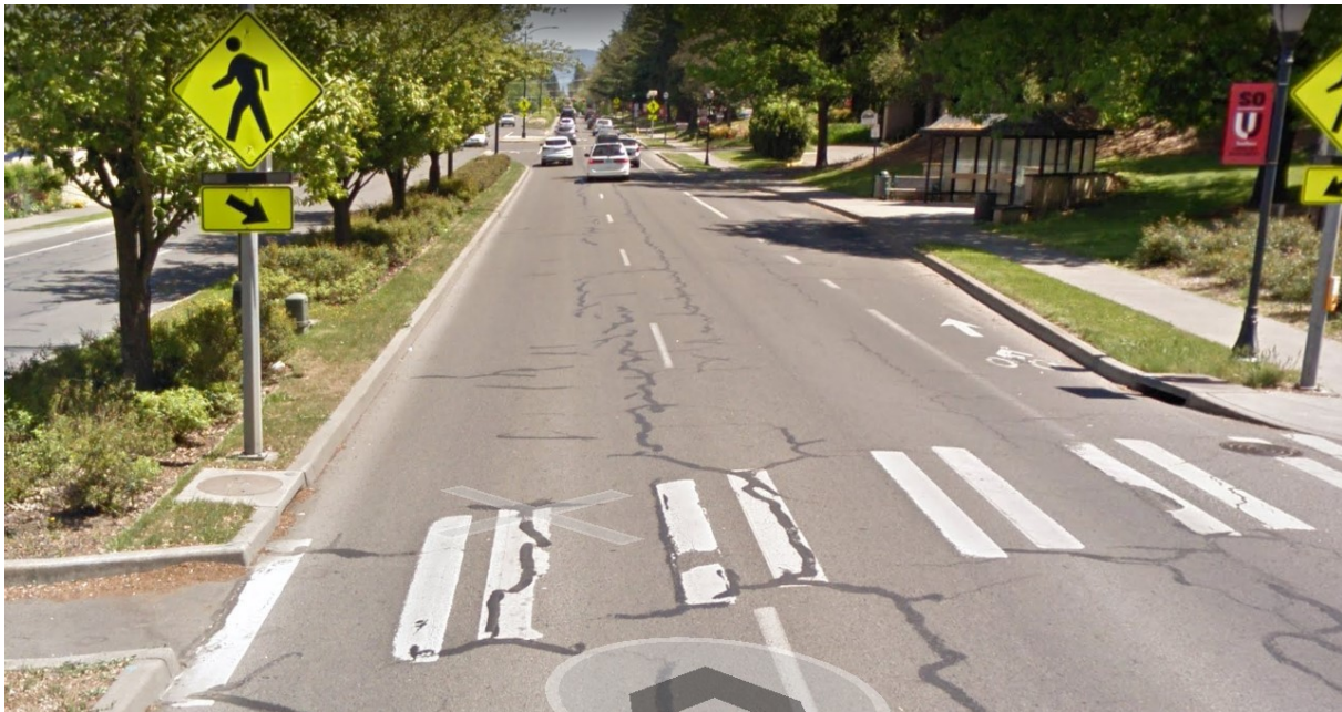
23 Figure 1 - RRFB at University Way
