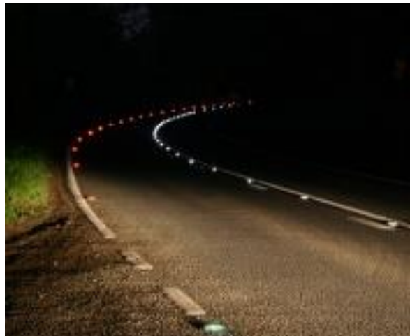
Fig 3. Solar Powered LED road studs. These are very reliable and offer an alternative solution to street lighting in areas where it is not appropriate. Credit: Astucia Traffic Safety Systems.
