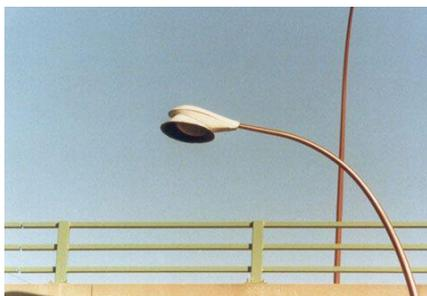
Figure 13 - Shielded Cobra Head<sup>21</sup>
