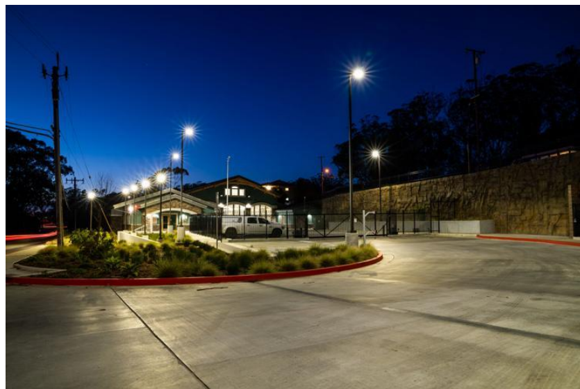
Figure 2 – El Granada Fire Station
