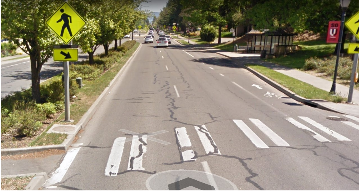
13 Figure 1 - RRFB at University Way
