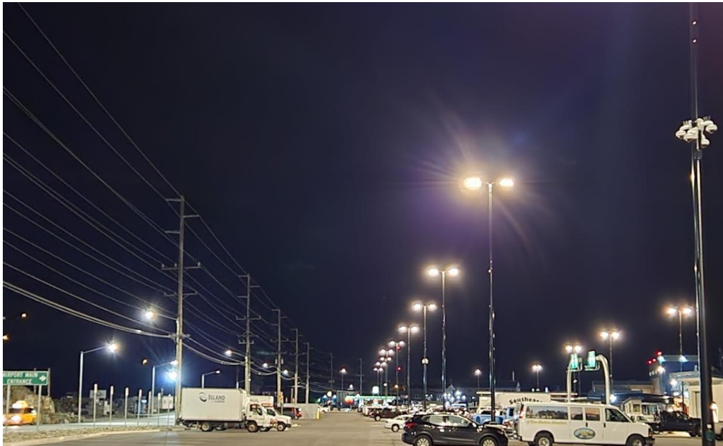
16 17 18 19 Figure 12 - LED Airport Lighting
