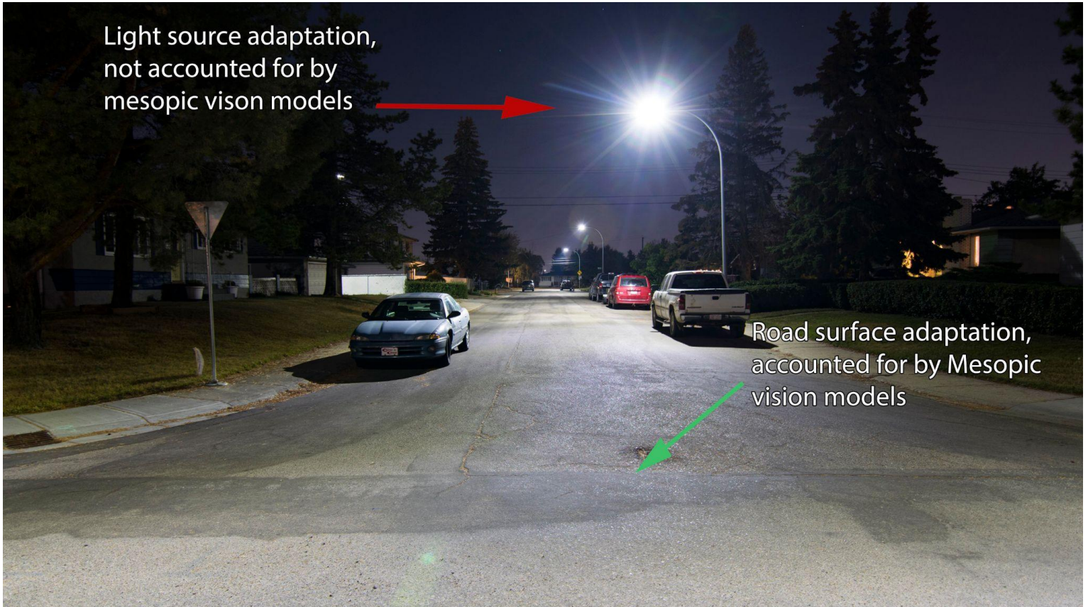
^Figure 4, A representation of visual field adaptation factors. Mesopic vision models such as MOVE and the Unified model only account for the luminance level of illuminated surfaces.
